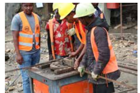
Workers at Thwake Dam construction site
